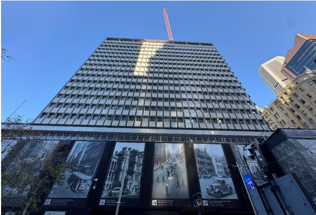
Figure 3: Site viewed from Martin Place
