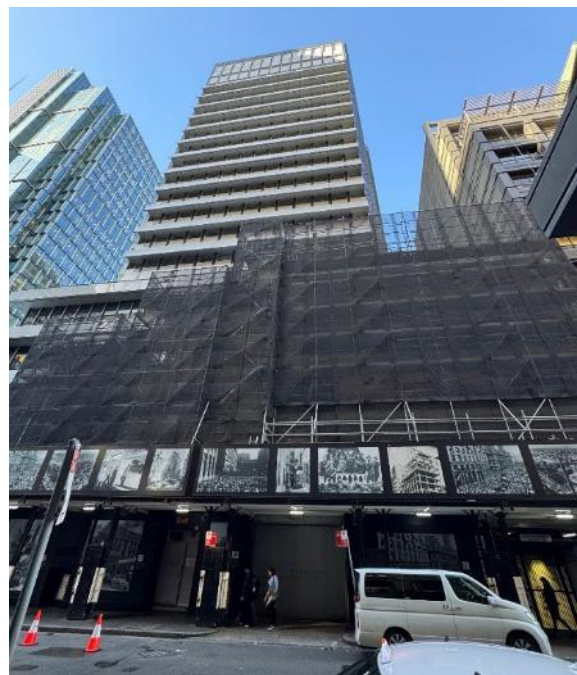
Figure 5: Site viewed from Philip Street
